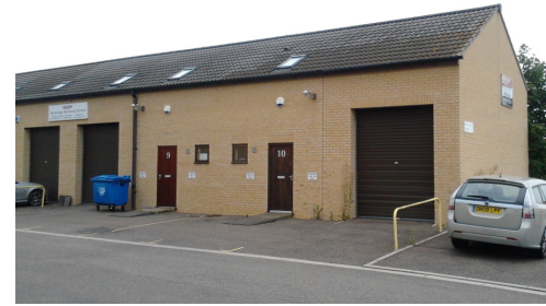
Example of modern small industrial unit.
